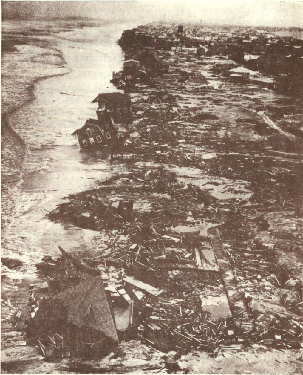
FIG. 1—Storm damage at Point O'Woods, Fire Island, N. Y., on March 7, 1962. (Photograph by United Press International.)
