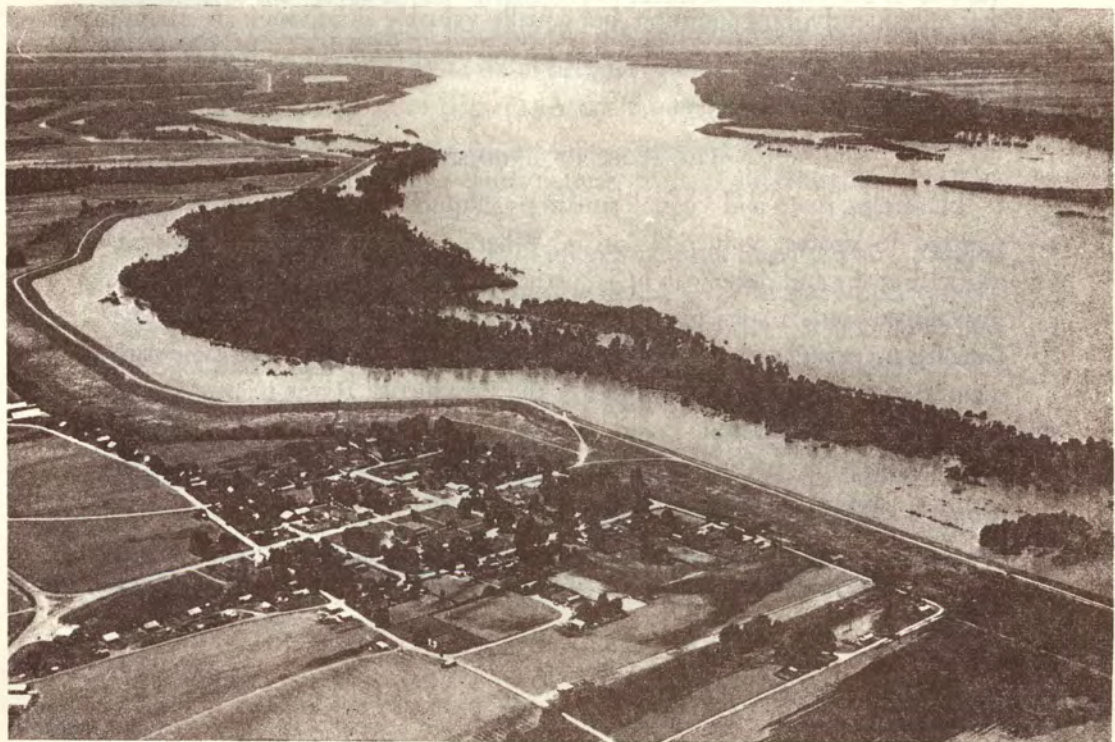
FIG. 8—A levee successfully holds back floodwaters of the Mississippi River on the wide floodplain of the Yazoo Basin, May 29, 1961. (Photograph by the U. S. Army Corps of Engineers.)
